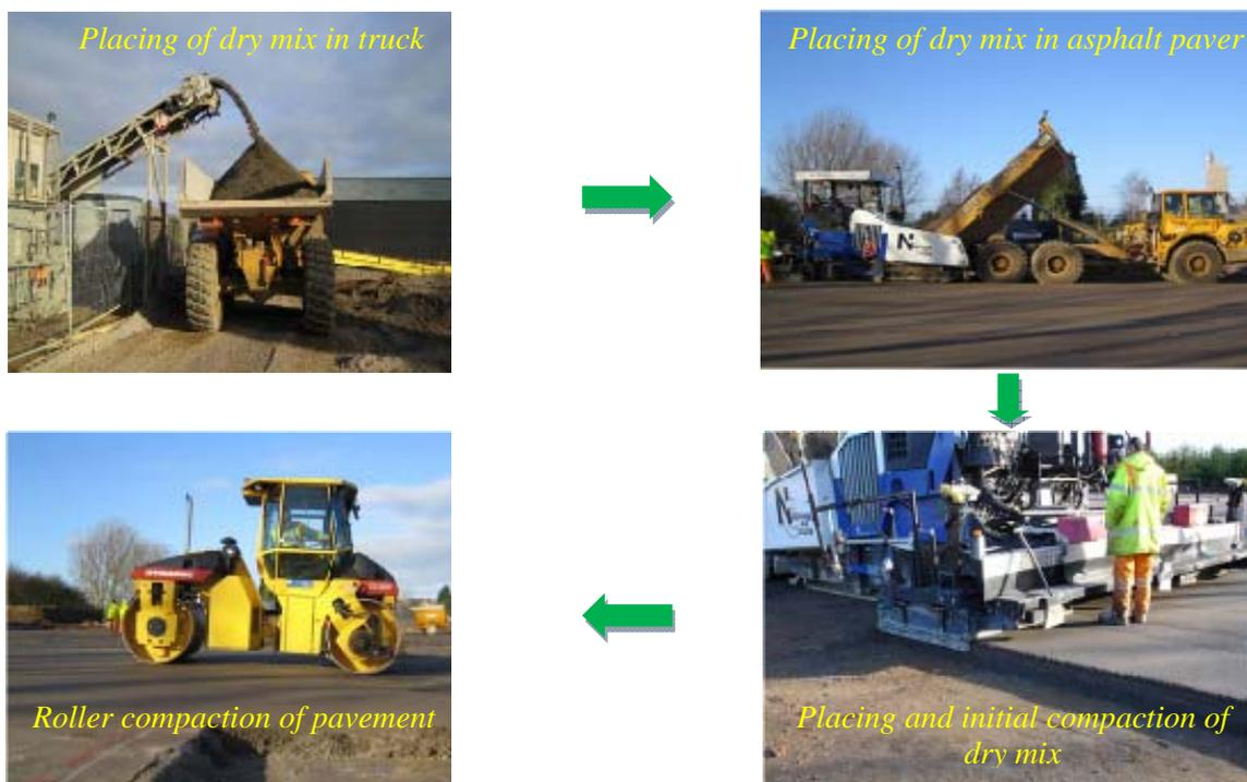
Figure 8 - Construction of roller-compacted plain-concrete pavements
