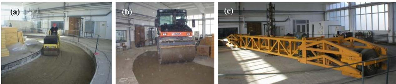
Figure 6 – (a and b) Construction of the trial SFRC sectors, ALT LIRA facility (c)
